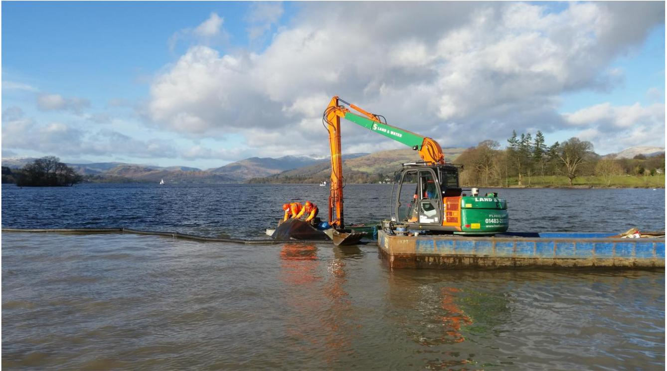
During the construction of the new **Windermere Jetty Museum of Boats, Steam & Stories** – where the Lakes Steam Boat Heritage is protected, a silt curtain was effectively deployed for 18 months to prevent contamination of Windermere whilst dredging and new quays were constructed. The museum opens late in 2017
