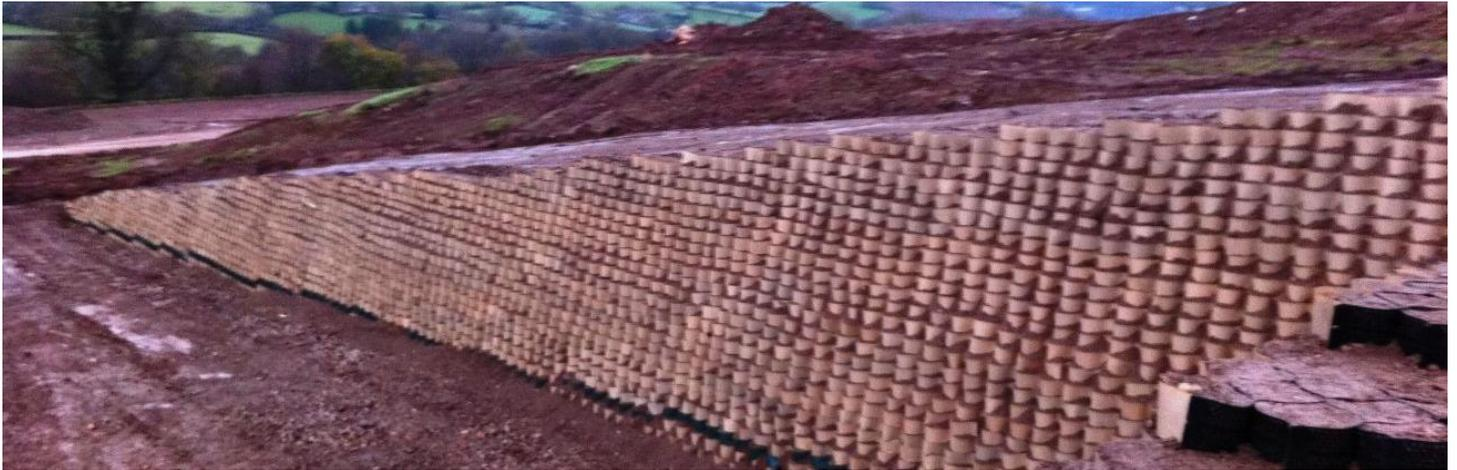
Provectus Remediation were looking for a cost-effective retaining wall solution that could be easily installed and landscaped. The Geoweb system allowed the use of onsite materials for infill and back-fill. Geoweb allowed reclamation of land areas with less than desirable soil properties. Topsoil in the outer wall fascia provided a natural environment for vegetation.
