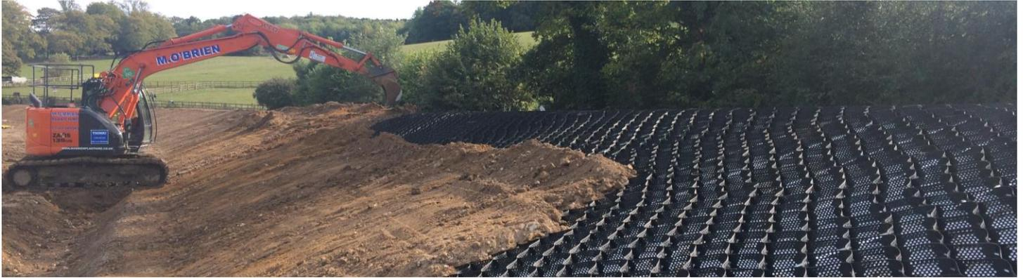
Following the catastrophic flooding of early 2014 temporary reservoirs were put in place to slow and divert the Caterham Bourne, an underground watercourse which had swollen following the excessive rainfall. During the summer more permanent defences were constructed comprising bunds surrounding storage areas for 10,000m<sup>3</sup> of water.
