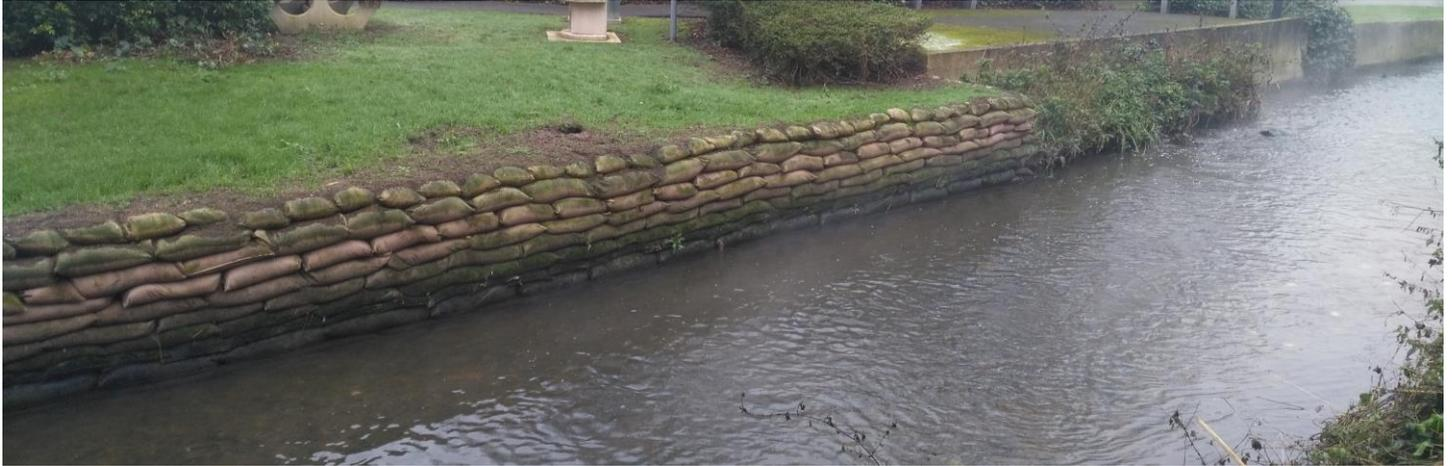
Following the discovery of instability in an embankment on the Hogsmill River in Kingston Upon Thames Surrey a solution to control further erosion of the island containing a hall of residence and The Stanley Picker Gallery was required. Due to the lack of vehicle access to site that solution had to be easy to transport and require a minimum of plant to install.
