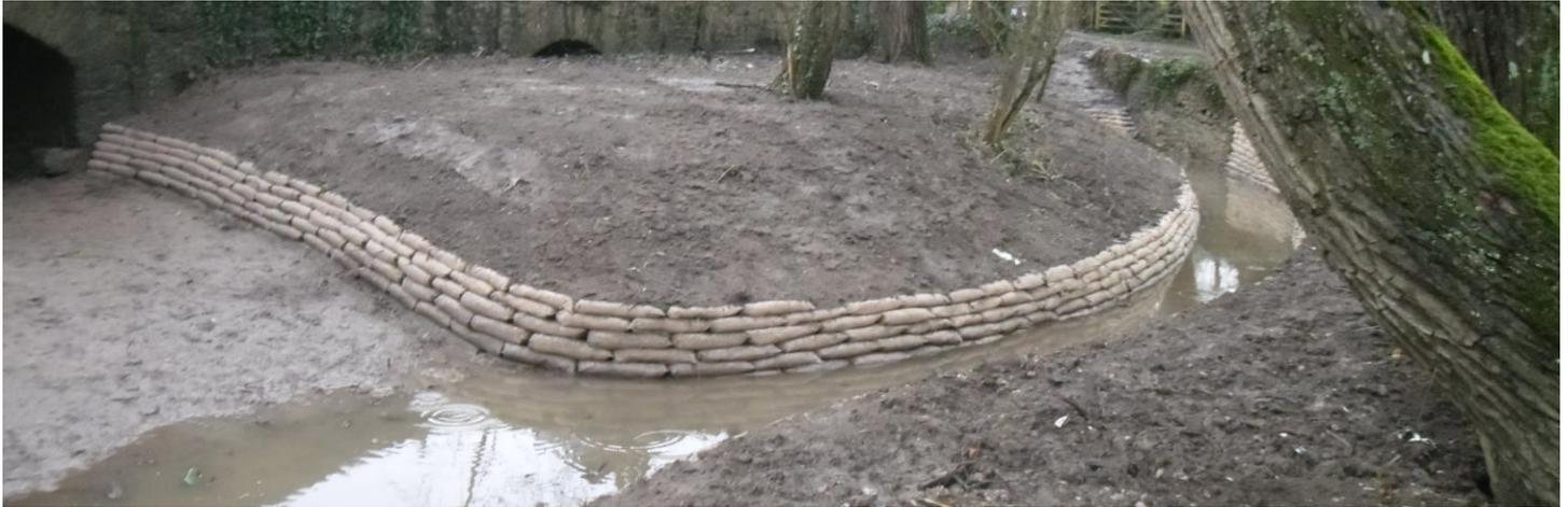
At this site in Rode, near Frome, increased water flow from the Mendip Hills was putting additional stress on the bridge that linked the village to the A36. The divert from the River Frome, which was originally created to form a mill race for Rode Mill, previously passed under one span of the bridge which now struggled with the increased water levels. Therefore, an additional channel was created to relieve this stress via a new pass under another span of the bridge during periods of high water.
