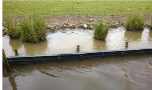
Nicospan has been designed specifically for vertical bank protection; it provides a proven and economical form of erosion control at the water edge. Nicospan is a prefabricated, double weave revetment fabric made from strong UV stabilised monofilament yarns that are heat sealed to form a series of open pockets so that 75mm $\phi$  - 100mm $\phi$  timber posts can be installed.
