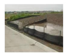
Greenfix 70SF Silt Fence is a temporary sediment control device used on construction sites to protect water quality in nearby streams, rivers, lakes and seas from sediment (loose soil) in storm water runoff. Silt-Stop 70SF is a high quality woven polypropylene geotextile made of 100% polypropylene staple fibres.
