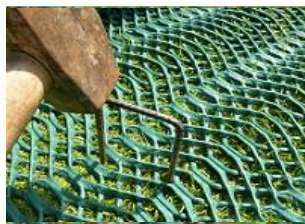
Fix using steel u-pins
