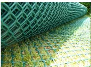
Unroll mesh onto existing grass
