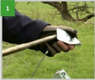
1 Insert Drive Rod into the Anchor
