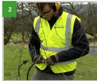
2 Thread guy wire through rubber sleeve
