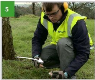
5 Thread guy wire through the second tensioner at ground level
