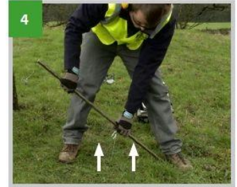
4 Activate Anchor by pulling the wire upwards
