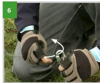
6 Loop guy wire through Quick Link
