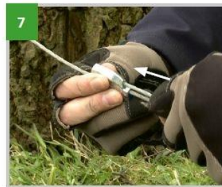
7 Create loop by putting tail through second tensioner
