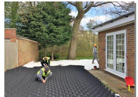
Geoweb® panels connected with Atra Keys® 3 times stronger and faster than staples
