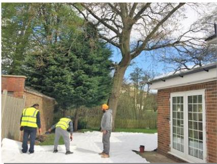
TRP 4000 Geotextile laid in TRP area to go under Geoweb®
