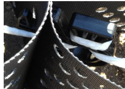
Figure 9 ATRA Tendon Clip secured with the Geoweb cell.
