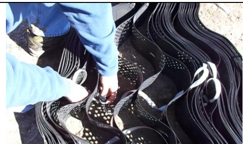
Figure 10 Preassembling ATRA Tendon Clips
