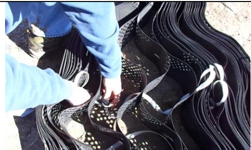
Figure 10 Preassembling ATRA Tendon Clips
