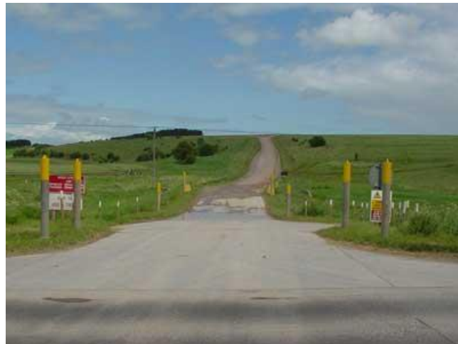
Typical section of Army road on Salisbury Plain, at an intersection with the public highway
