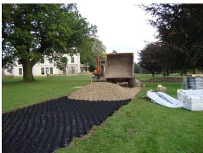
Only 200mm of subgrade was excavated compared to the 500mm required for conventional road construction and subgrades of this CBR value. TRP3000 300gsm needle punched geotextile was laid to provide a suitable separation layer between the subgrade and the specified aggregate. This grade of geotextile was selected to give the best compromise between infiltration of water from the permeable surface to the subgrade, and the strength required for the load support system to perform as expected.
