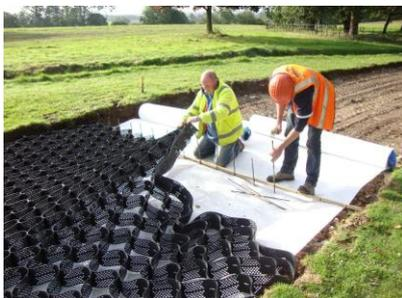
Without proper support areas used by traffic will rapidly deteriorate to a point where they become unusable. The relatively poor soil of the local area means that using Geoweb reduced excavation and aggregate requirements while minimising the likelihood of settlement and deformation.
