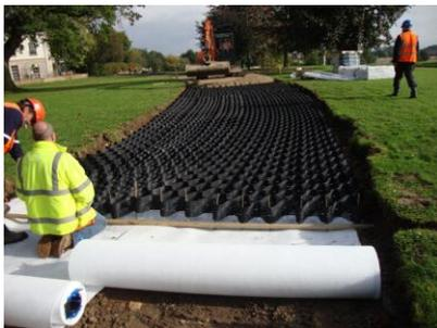
Copt Hewick Hall is a privately owned grade II listed building near Ripon, North Yorkshire. As part of an extensive renovation a service road was created using 150mm deep Geoweb. With a permeable surface such as that being used on this site confining the aggregate within the cells Geoweb improves the load distribution characteristics, reducing long term maintenance requirements.
