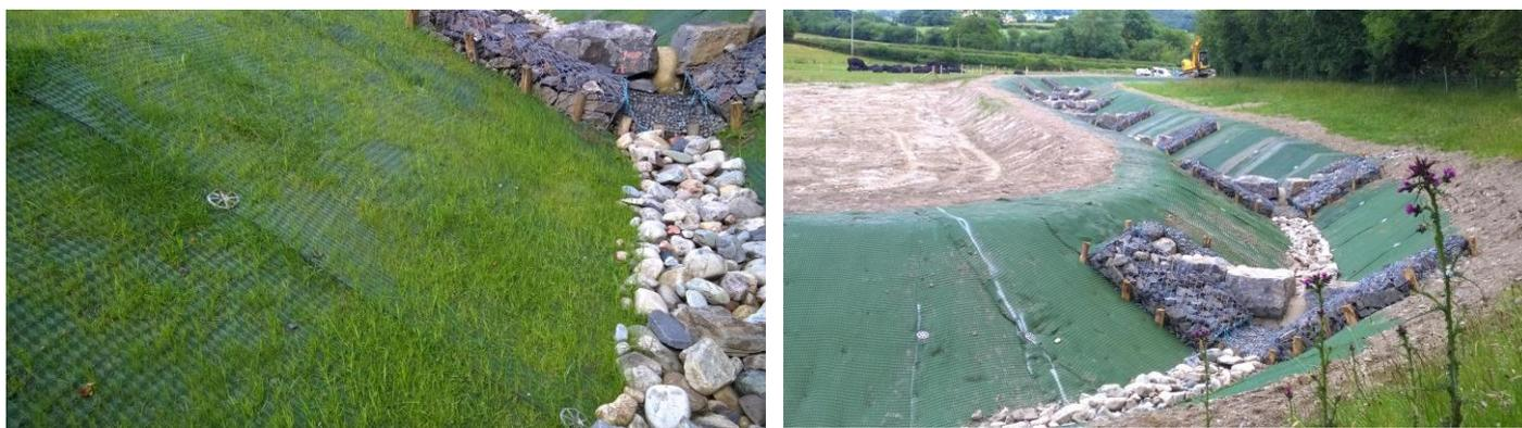
The completed PP5-Heavy Duty slope provides a secure surface once fully established and the permanent nature of the matting coupled with the Greenfix Anchor System ensures long term turf reinforcement and the immediate erosion control required by the constantly flowing water of the fish pass.
