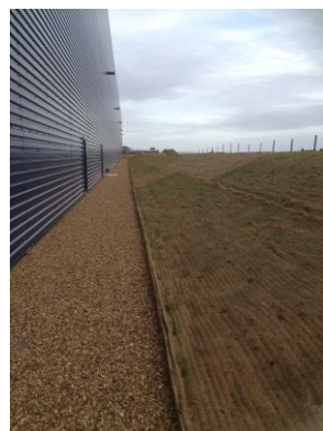
Matting installation completed
