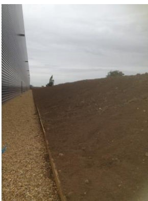
Slope raked level prior to installation
